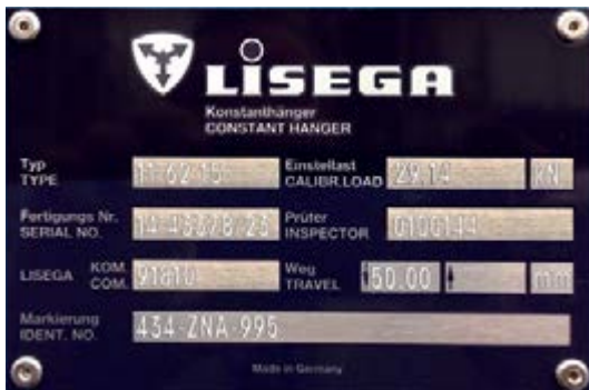
Name plate with stamped operating data
