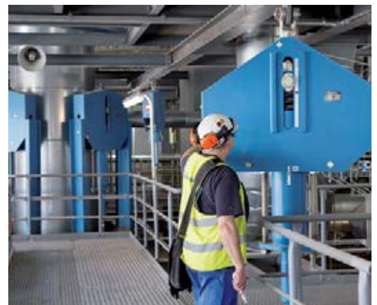
Installation inspection of a constant hanger
